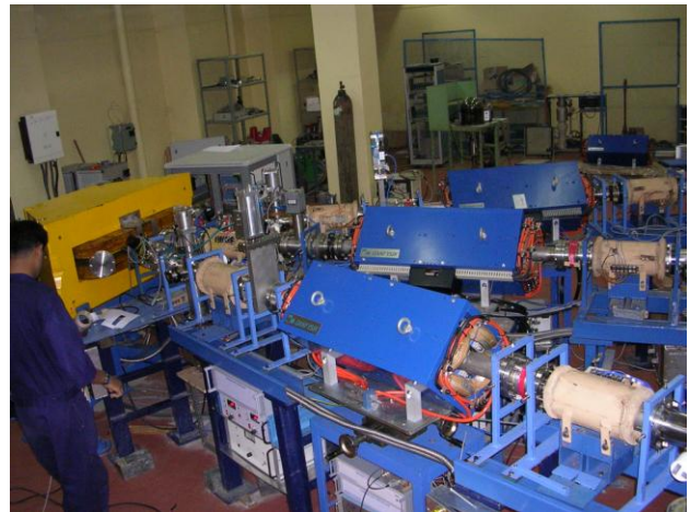
Figure 5: 5-port Switching Magnet and beam lines
