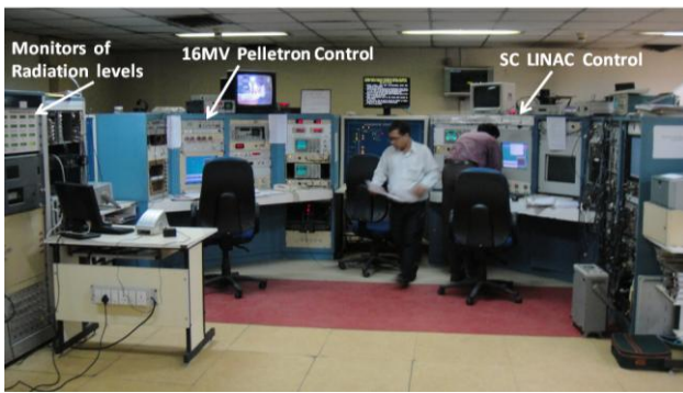
Figure 5. Control Room for 15UD Pelletron and superconducting LINAC.
