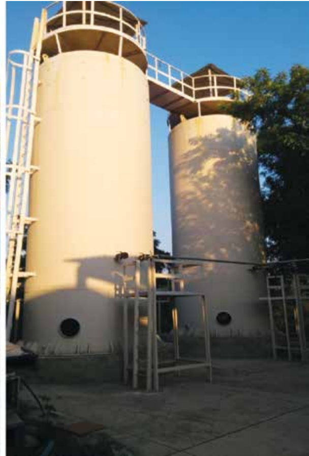
Fig. 3.1.8: 2x60 M 3 new helium gas tanks
