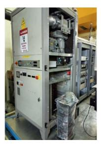
Figure 2.6: Klystron along with the repaired Servo stabilizer.
